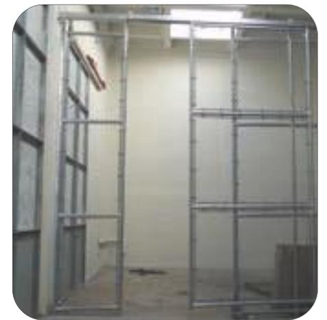
*Specially-constructed slide gates are fitted to the interior holding pens of the giraffe night house. There are three total, and they are 15-ft. tall with 3-ft. openings, mounted on overhead tracks. A special stainless steel pull rod was attached to each gate to allow the keeper to open it from a secure area. The giraffe pens were built from chain link ranging from 42-in. to 17-ft. in height.*
