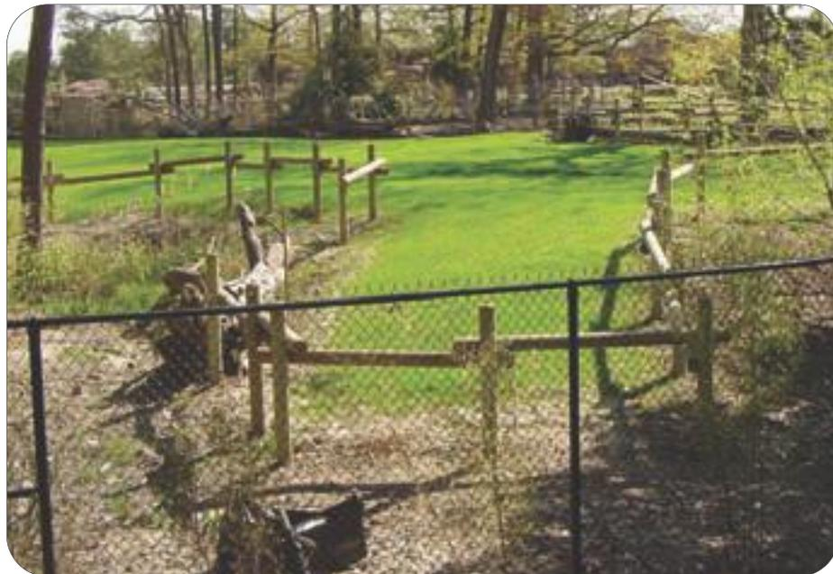
*At left is another view of the giraffe restraint fence showing the chain link and post and rail portions. Above, elephants are restrained by this heavy-duty gate constructed of 6 5/8-in. horizontal, diagonal and vertical rails, all coped and welded. The posts are 6-in. wide flange beams set 8-ft. into the ground, with the gate swinging on custom hinges. The gates are 8-ft. tall and 13-ft. wide. Below, a detail of a rhino/zebra swing gate. (Hercules Fence photos)*
