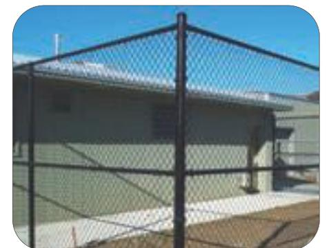
*The zebra pens were fabricated from black vinyl coated chain link on vinyl coated framework with top and mid rail. Below is the slide gate through which zebras and rhinos pass.*
