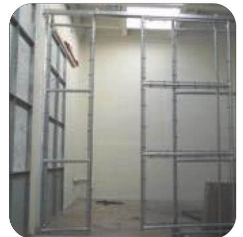
*Specially-constructed slide gates are fitted to the interior holding pens of the giraffe night house. There are three total, and they are 15-ft. tall with 3-ft. openings, mounted on overhead tracks. A special stainless steel pull rod was attached to each gate to allow the keeper to open it from a secure area. The giraffe pens were built from chain link ranging from 42-in. to 17-ft. in height.*
